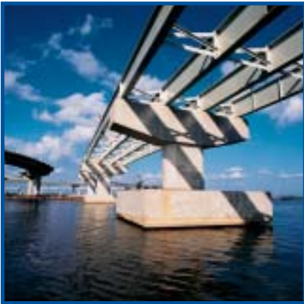
Bridge during construction.
