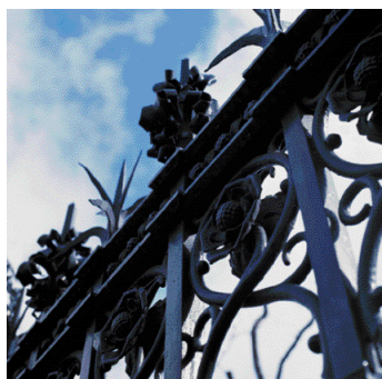
Bare wrought iron can begin to rust in just a day or two.
